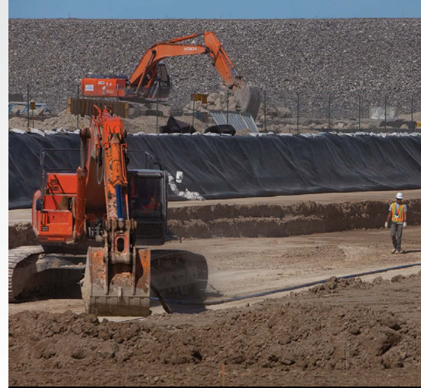
Clive Disposal Facility
