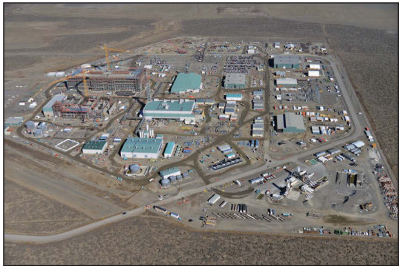
Technical issues have delayed the completion of Hanford's Waste Treatment and Immobilization Plant, known as the Vit Plant. (Photo: DOE/BNI)
