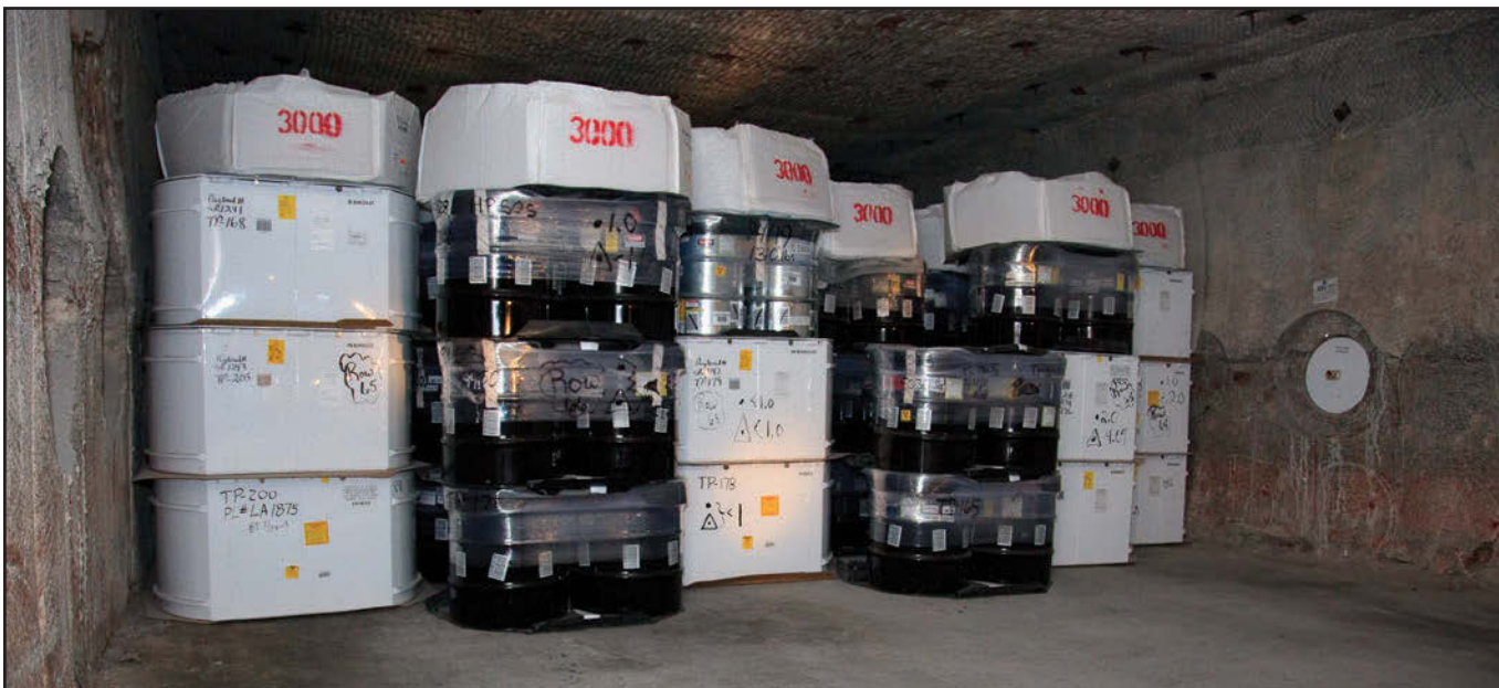
Waste handling operations at the Waste Isolation Pilot Plant were briefly suspended in May due to a misaligned waste container. (Photo: DOE)
