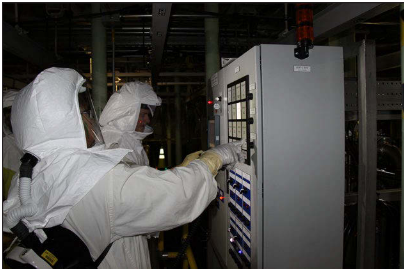
Workers operate a sludge removal equipment control panel during the transfer of the mixture out of Hanford's 105-K West Basin. (Photo: DOE)
