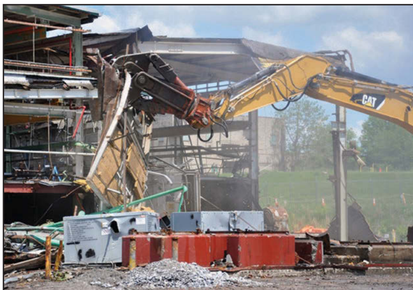
Crews began tearing down the K-633 Test Loop Facility at the DOE's Oak Ridge Reservation in May and completed the project in June. (Photo: DOE)
