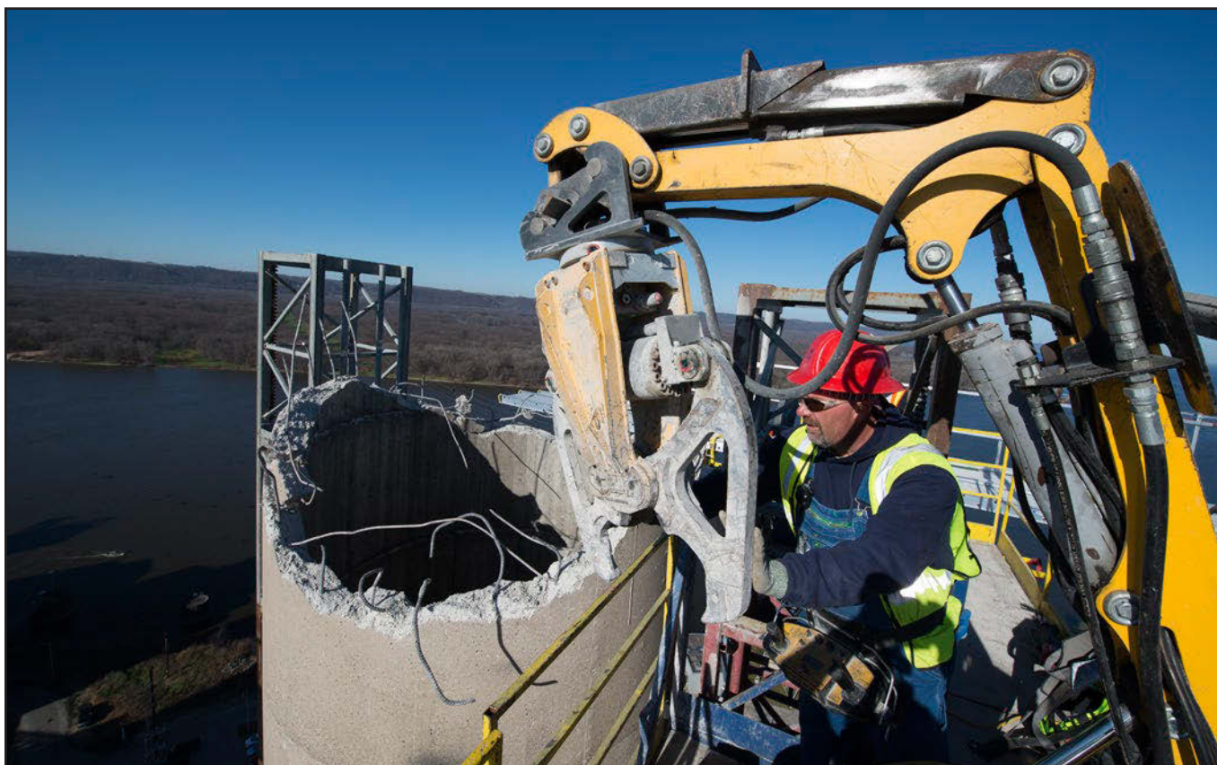
In 2016, EnergySolutions took operational control of LACBWR, allowing the company—as the 10 CFR Part 50 licensee—to continue expedited decommissioning activities at the plant. Demolition of LACBWR is expected to be completed in 2018. Removal of the plant's 350-foot-tall ventilation stack took about 150 days.
