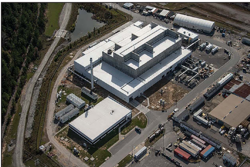
The Savannah River Site's Salt Waste Processing Facility is currently undergoing testing and commissioning. (Photo: DOE)
