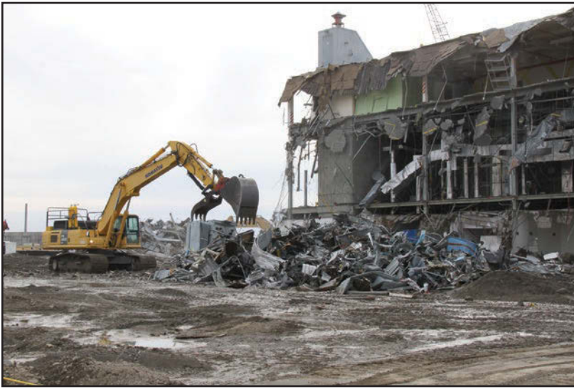
Demolition of Hanford's Plutonium Finishing Plant has been on hold since December 2017, when contamination was found outside the demolition zone. (Photo: DOE)
