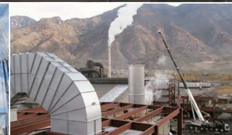
Pacific States Cast Iron Pipe Plant Modification
