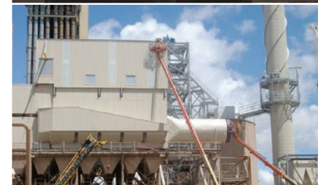
Solios/Ashgrove Cement Plant Modification
