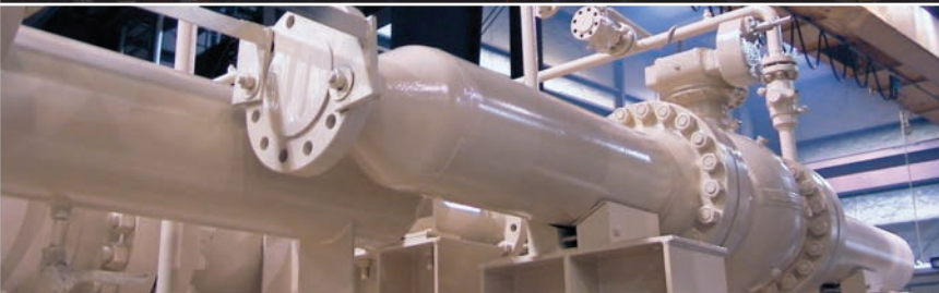
Skid Mounted Pipe Spools
