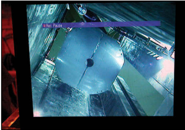
In this underwater view, a transfer cask is seen being lowered into the reactor's cask pit.
