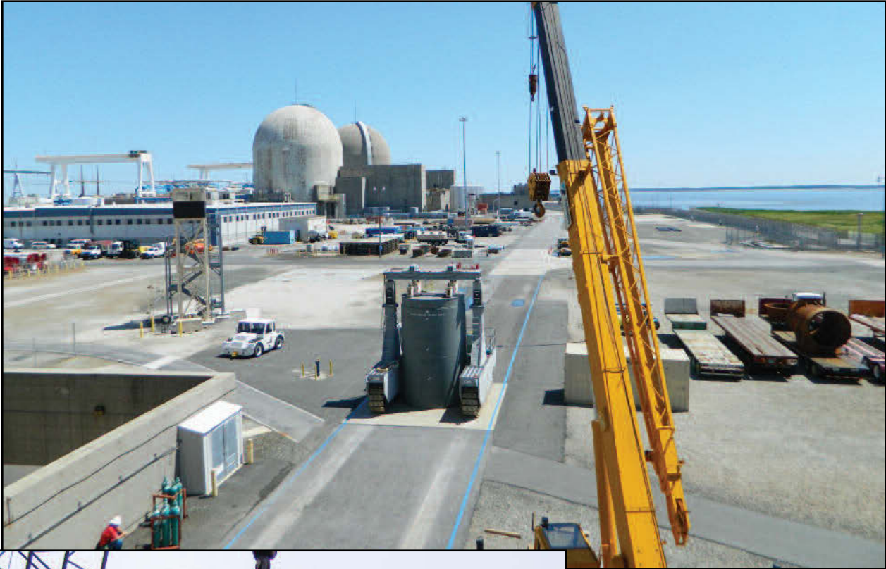
Above: Using a VCT, the cask is moved to the plant's ISFSI for long-term storage.
