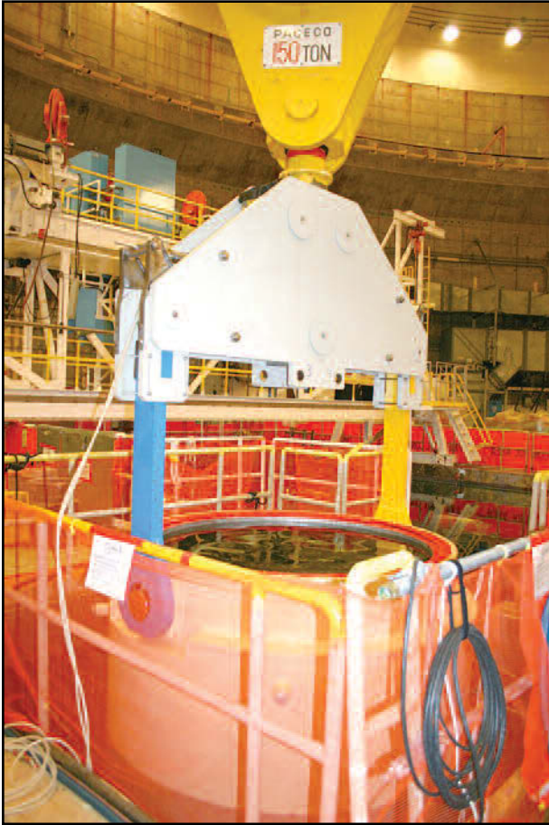
A HI-TRAC transfer cask is moved into the cask pit for loading used reactor fuel.
