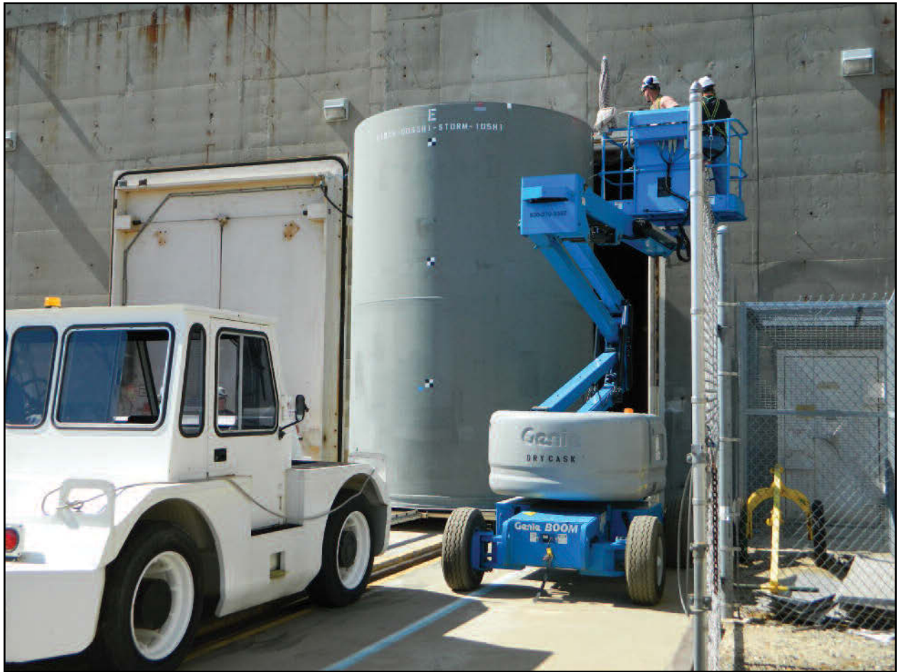
An empty Holtec HI-STORM dry storage cask is moved into the truck bay at PSEG Nuclear's Hope Creek nuclear power plant in Salem, N.J. (Photos courtesy of PSEG Nuclear).
