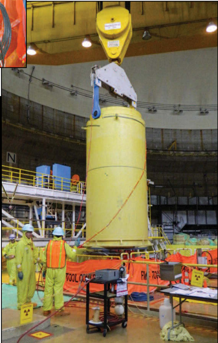
The loaded transfer cask is raised out of the cask pit.
