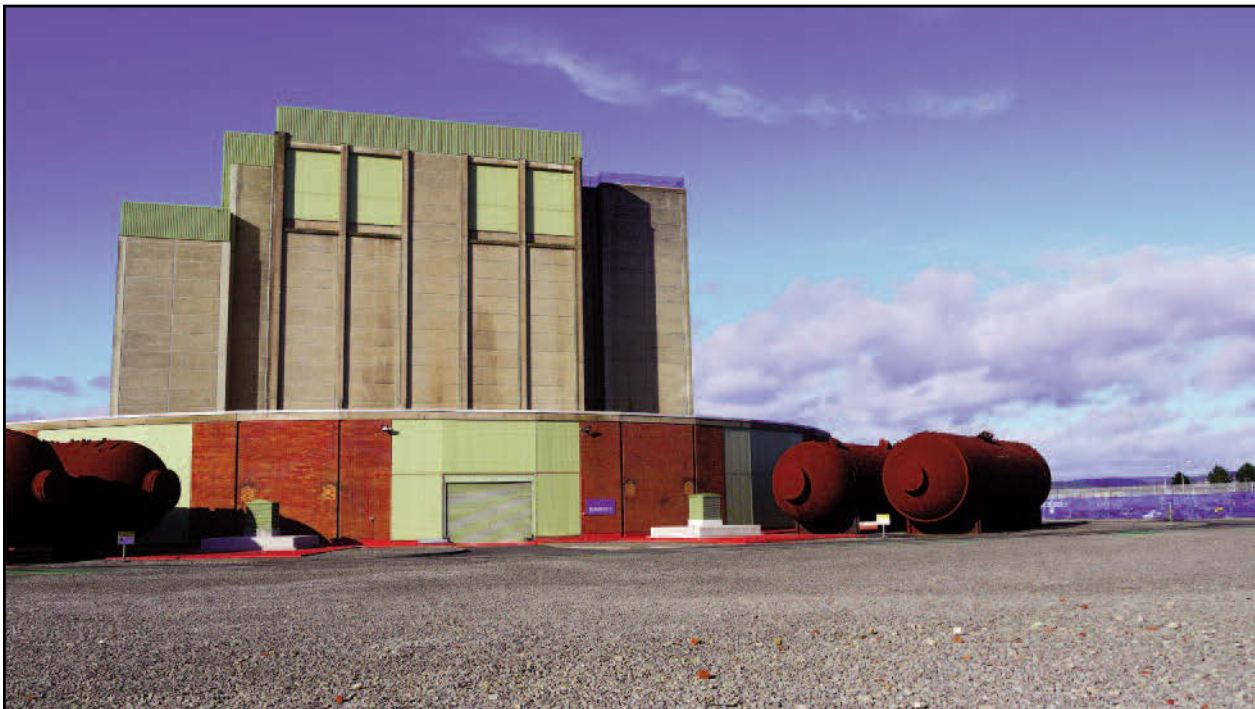
Fig. 2. Unit 1 at the Berkeley nuclear power station in safe storage condition, with the boilers shown stored horizontally next to the reactor building. (Photo: Magnox Ltd./www.magnoxsites.com)
