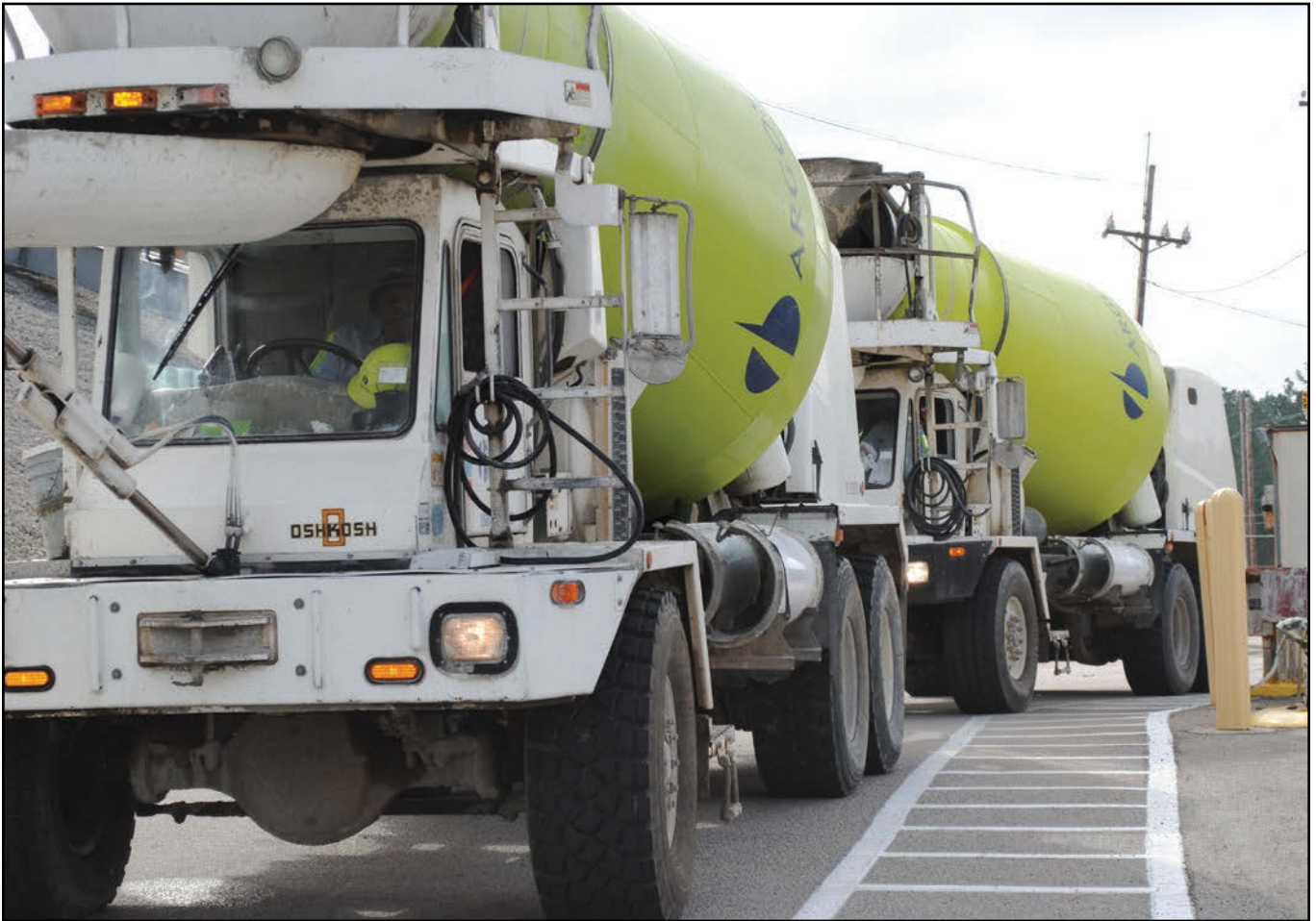
Cement trucks line up on June 2, 2015, to begin filling Tank 16 with specially formulated grout.
