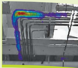
Hot spot detection while surveying piping
