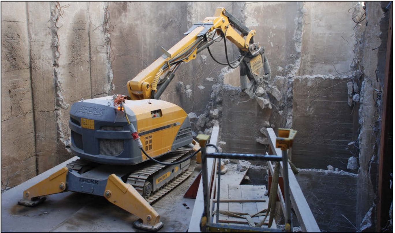
Fig. 2. A Brokk 330 demolition robot with concrete crusher attachment. (Photo courtesy of Brokk)
