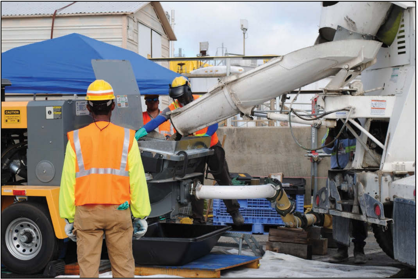
A cement truck begins the initial pouring of grout into Tank 16 at the Savannah River Site on June 2.
