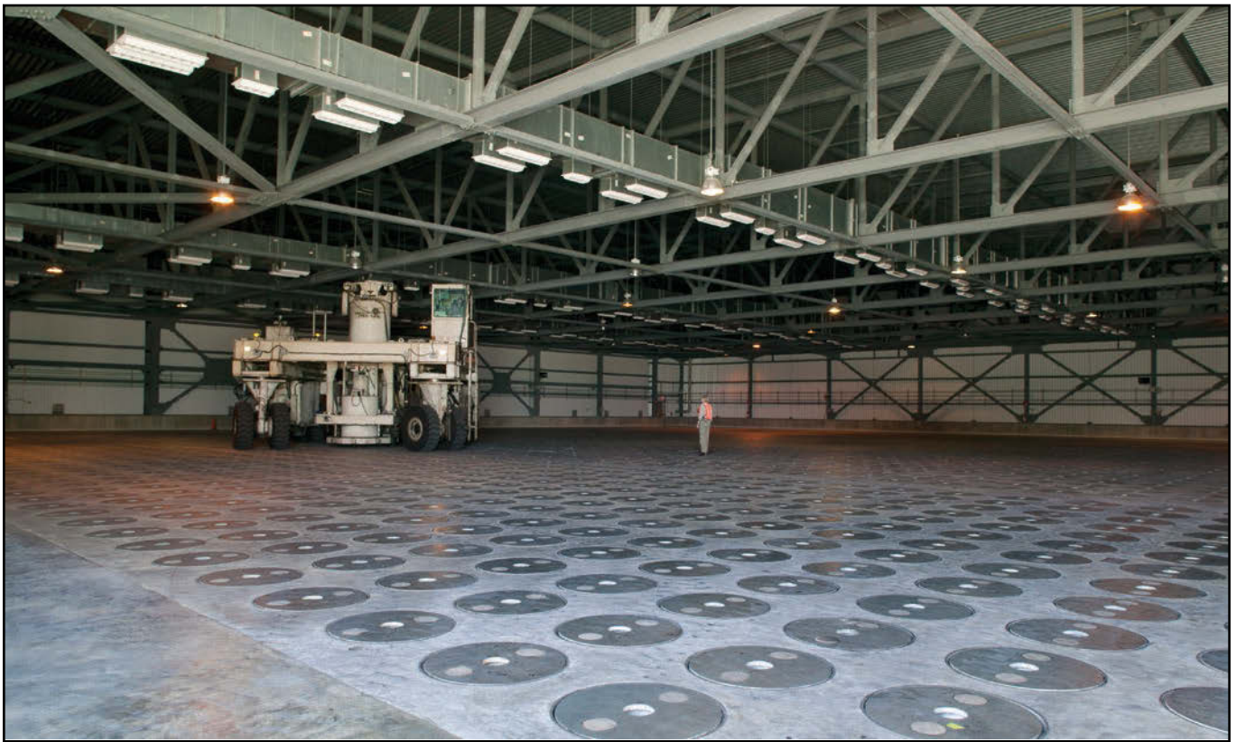
Glass Waste Storage Building 1 at SRS is the interim storage facility for vitrified waste after being treated at the DWPF. The vehicle, called the shielded canister transporter, transports canisters one-by-one from DWPF to the Glass Waste Storage Buildings.
