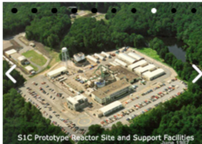
S1C Prototype Reactor Site and Support Facilities
